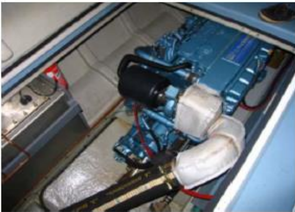
Port Engine Room
